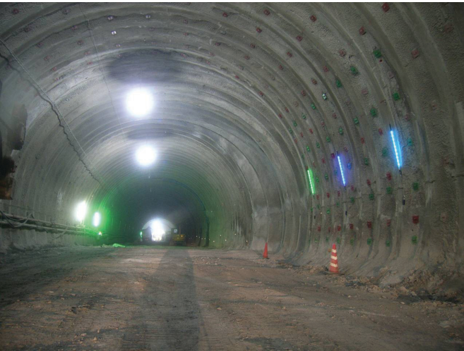
Figure 2. Visualizing convergence displacement of a tunnel. (Picture courtesy of Nexco East and Konoike Construction).
