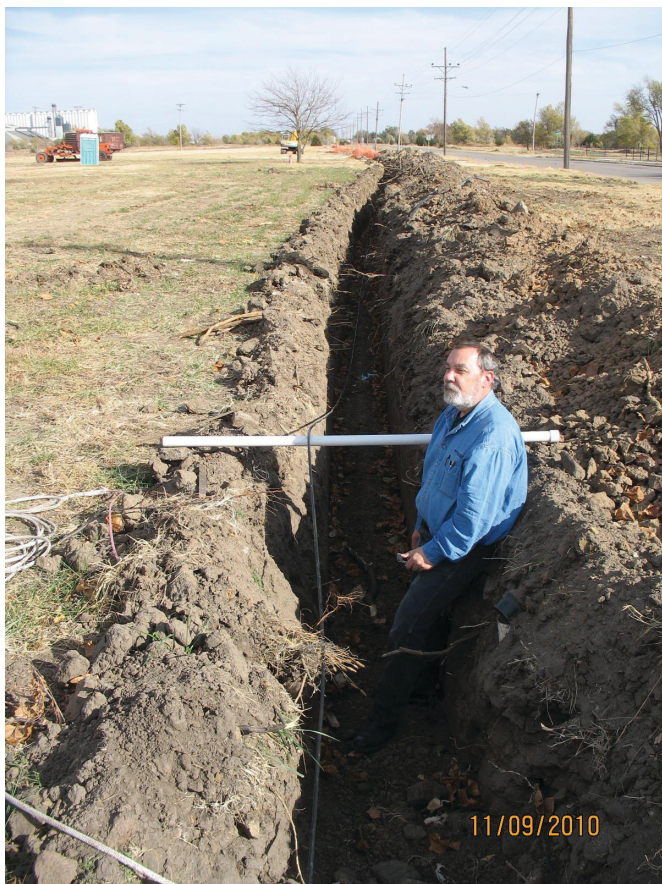
Figure 5. Site pull test.
