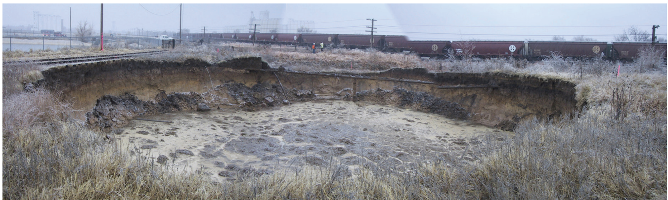
Figure 1. Sinkhole formed rapidly in 2005, at Old Brine Well at the Hutchinson site.
